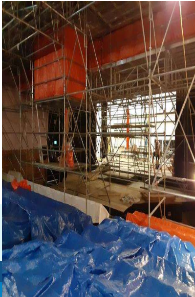
Auditorium - abatement and seismic reinforcement of the structure
