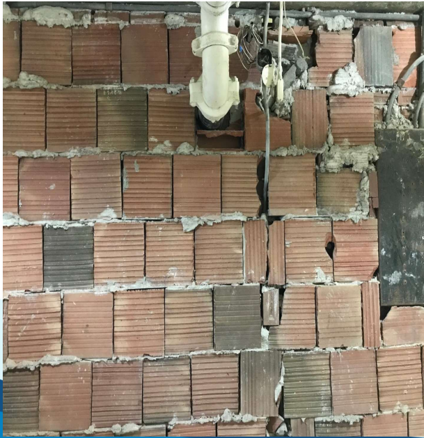
Unreinforced Clay Tile Wall
