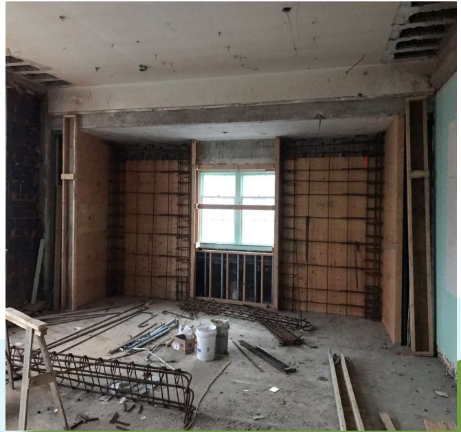
New reinforced concrete shear walls
