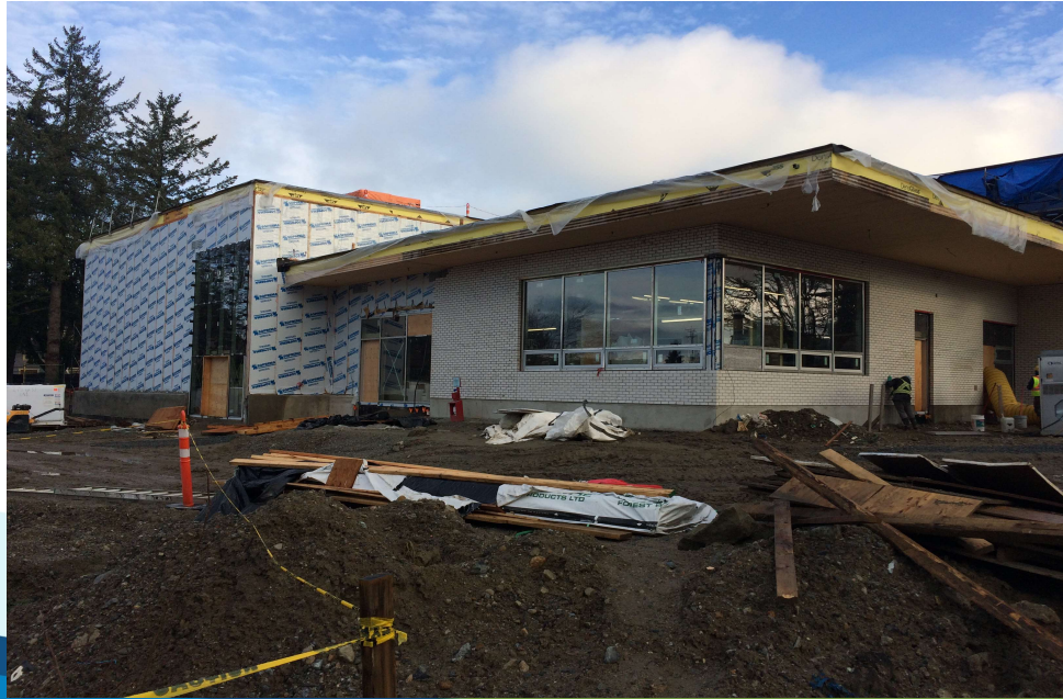
Exterior view of multipurpose room and gym
