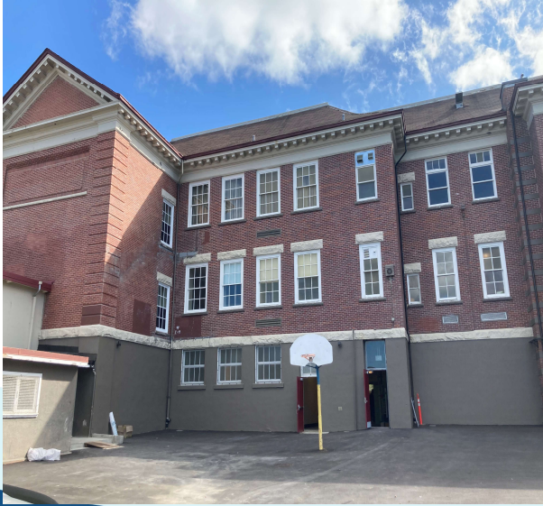
West façade of the school
