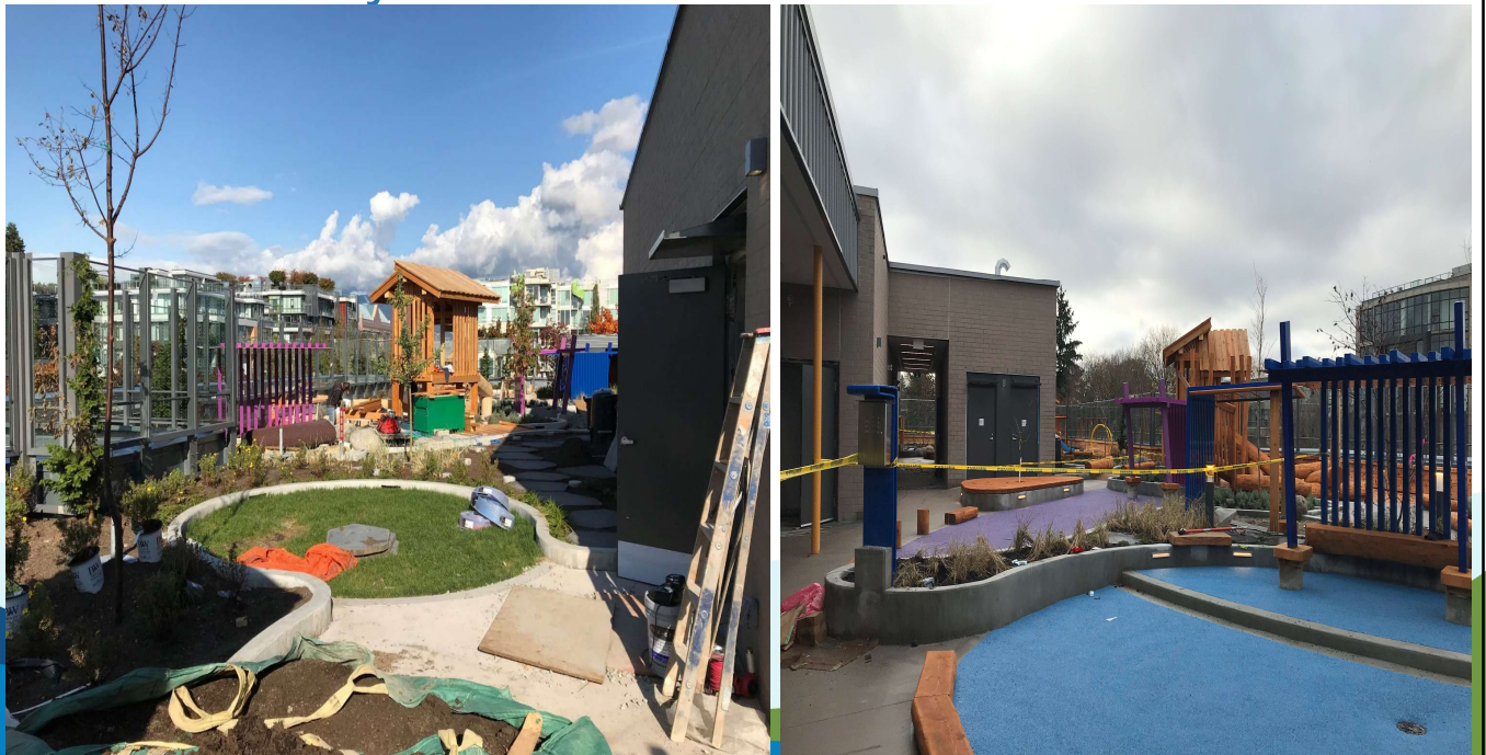
Rooftop Childcare Play Area
