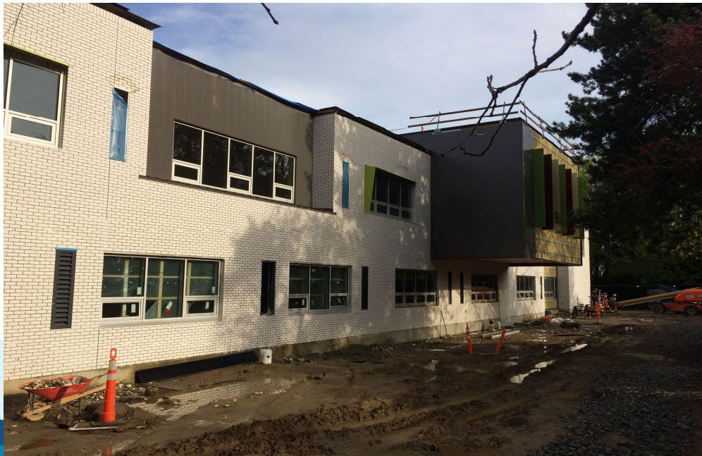
Exterior view of east elevation classroom blocks
